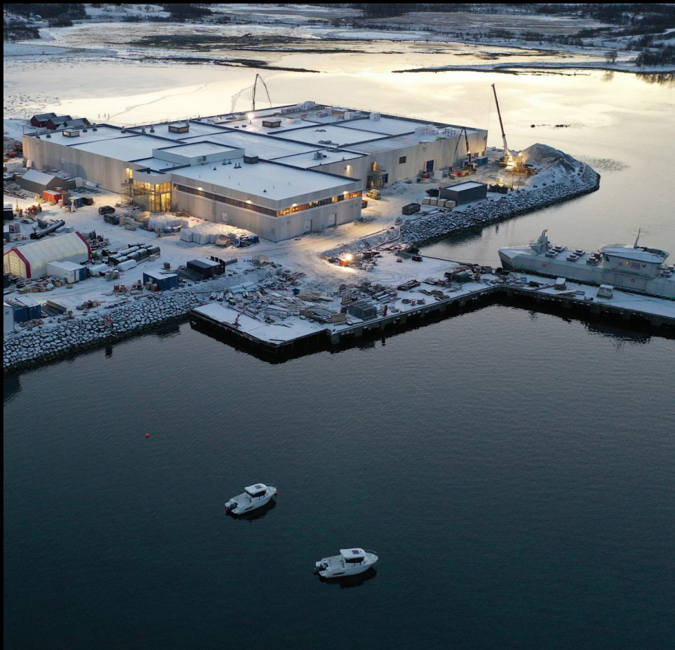
Norway Royal Salmon - Dåfjord, smoltanlegg, Troms, ferdigstilt i 2021
